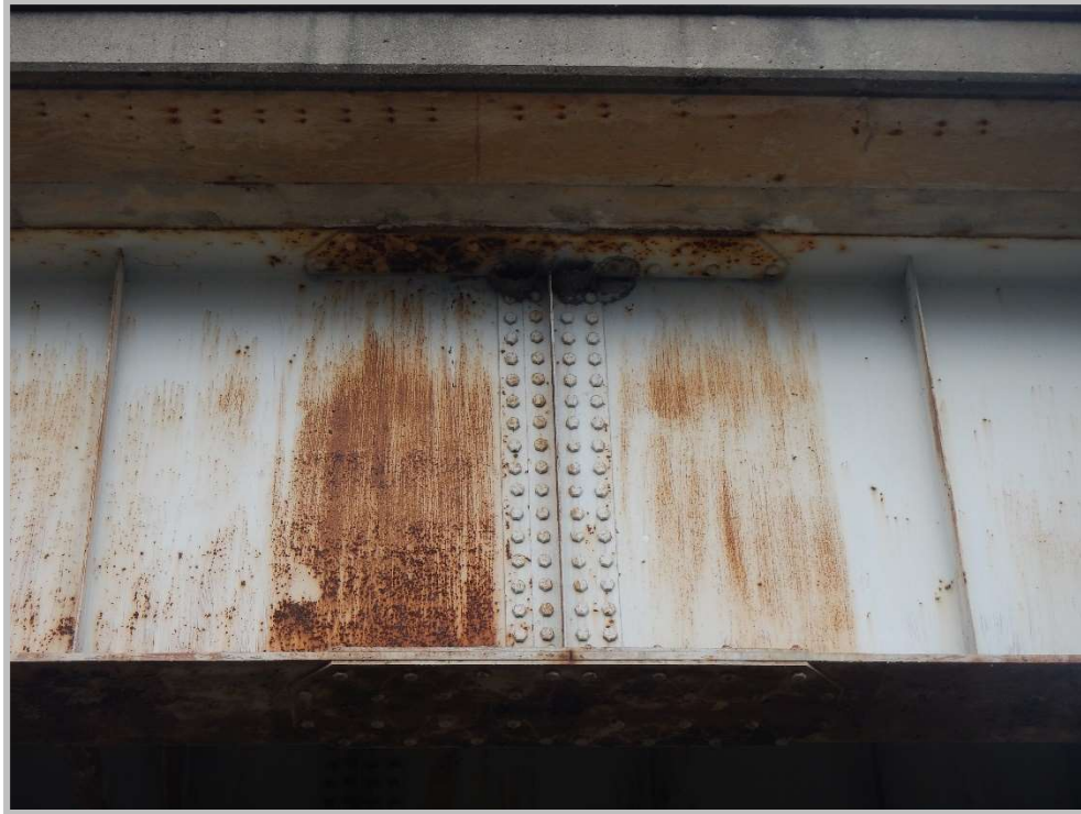
STEEL GIRDER BOLTED SPLICE AND TRANSVERSE STIFFENER
