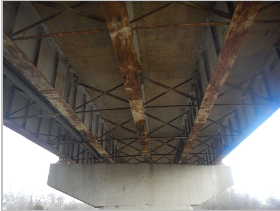
BRIDGE UNDERSIDE AND PIER CAP
