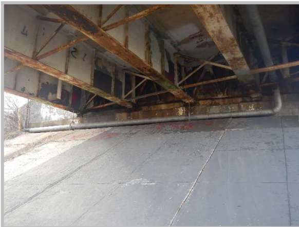
REAR ABUTMENT ELEVATION VIEW
