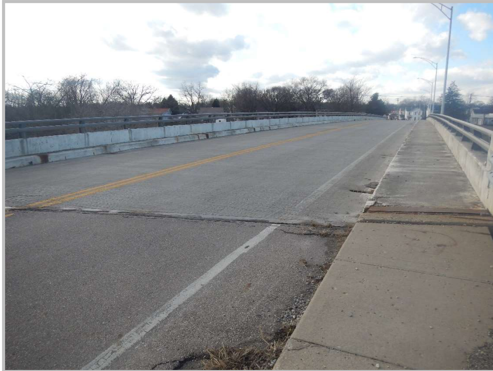
TOP OF THE DECK, SIDEWALK, SCUPPERS, AND APPROACH SLAB
